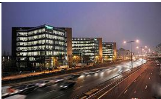
Schneider Electric head office in Paris
