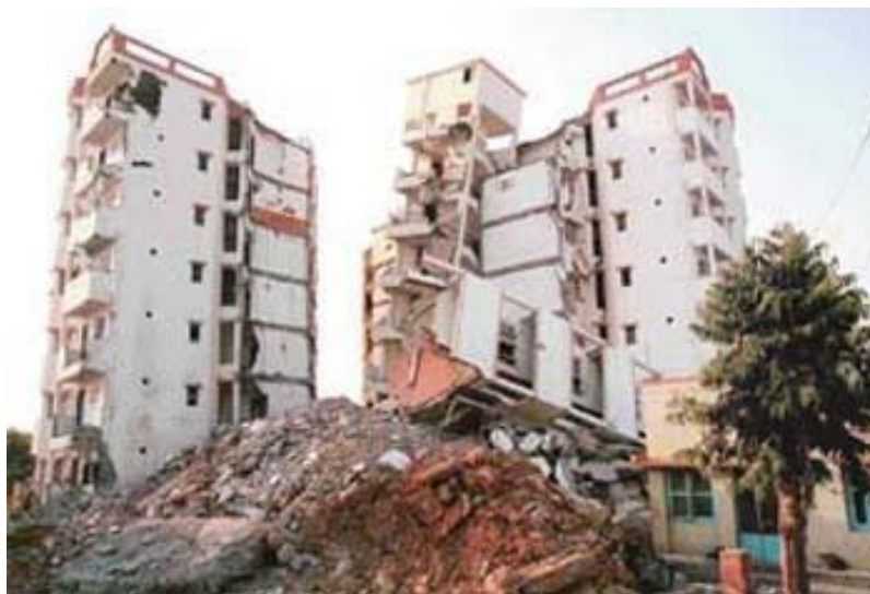
Fig. 2 Effect of Bhuj earthquake on building
