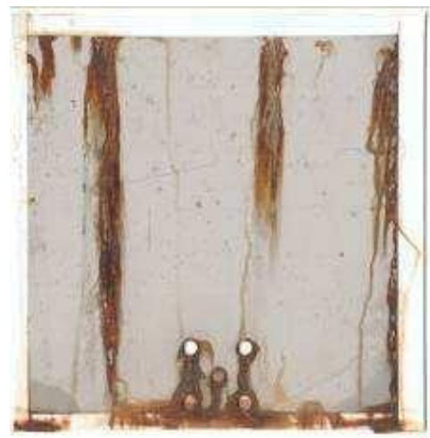
Figure. 6.10: Bad adhesive tape can lead to corrosion
