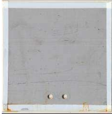
Figure. 6.11: Good adhesive tape can avoid corrosion
