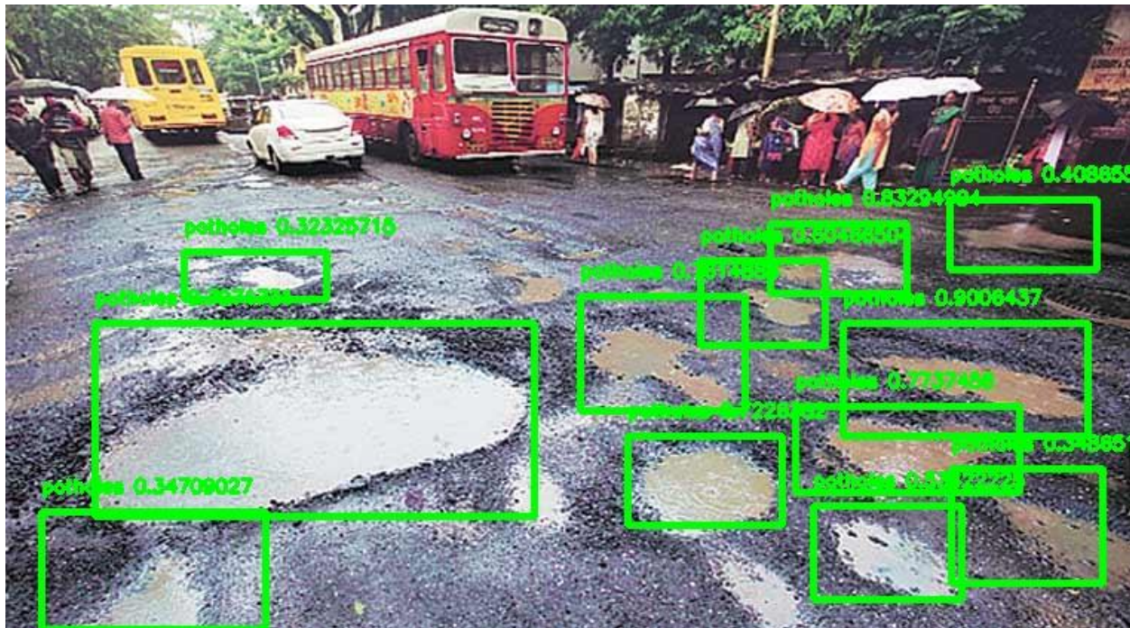
Fig 7.1 Tested pothole image
