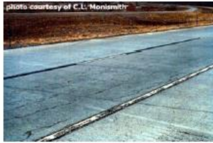
Shrinkage cracking
