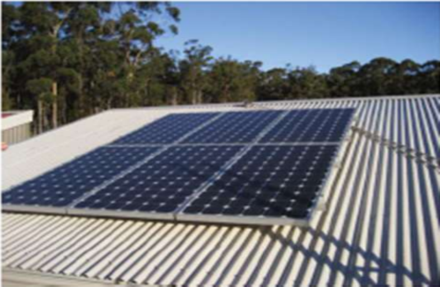
Figure 4.22 Even this small shadow can reduce the amount of electricity a module produces – a small shaded area can, under certain circumstances reduce module output by 80–90 per cent as well as affecting the rest of the array
