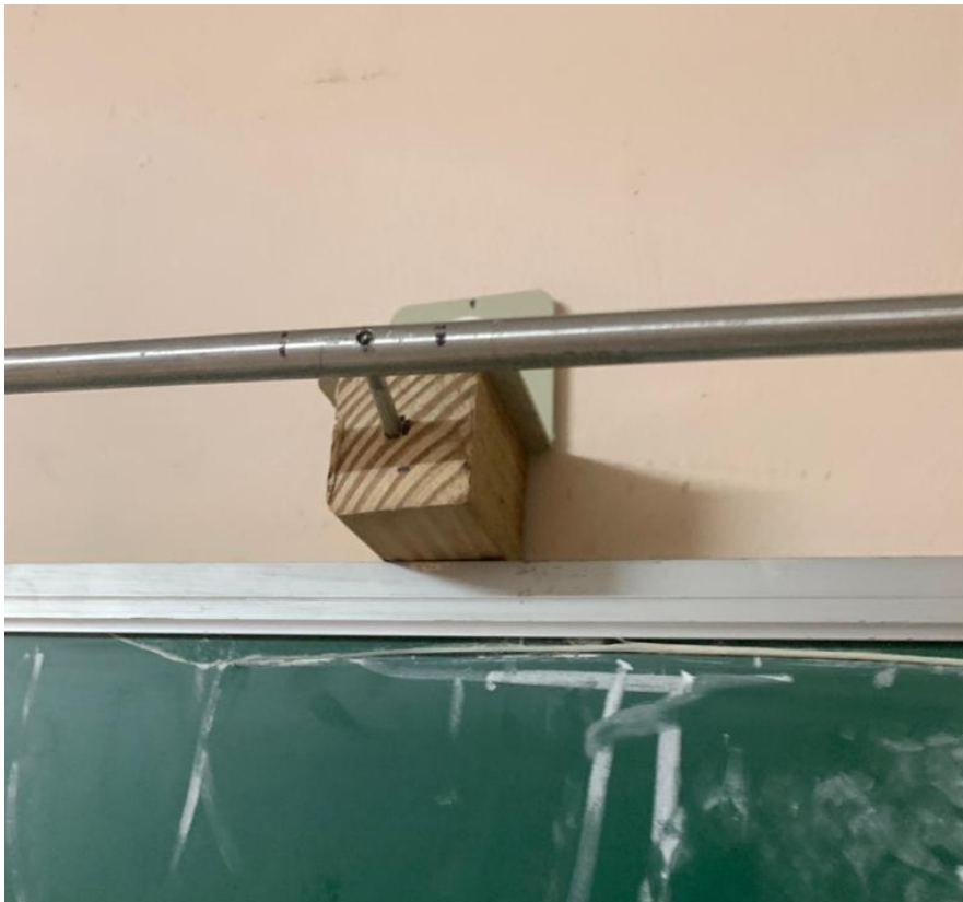
Fig 15: Upper rod center support
