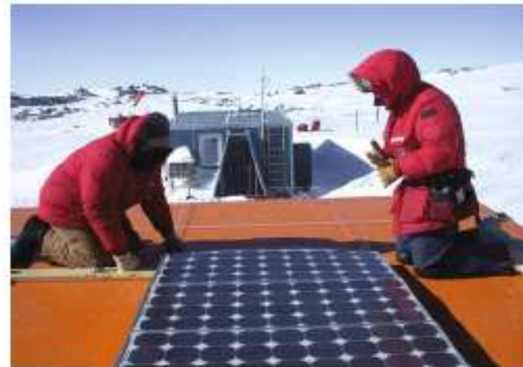
Figure 4.20 PV modules perform well in cold and sunny areas. They are often used as a power source in Antarctica during the summer. However, because there is so little light in winter, diesel generators are typically used as back-up.
