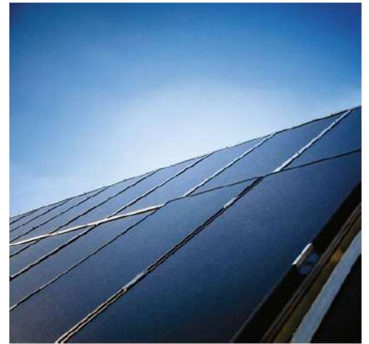
Figure 3.5 Amorphous silicon modules are easily distinguished from crystalline modules by their dark and uniform colour but they also look like non-silicone thin film modules
