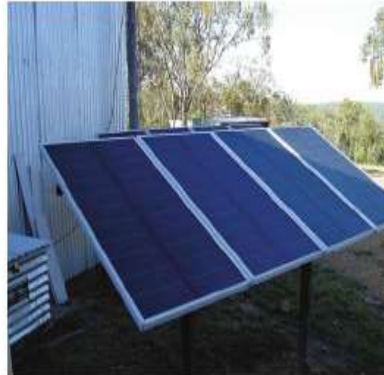
Figure 4.22 Even this small shadow can reduce the amount of electricity a module produces – a small shaded area can, under certain circumstances reduce module output by 80–90 per cent as well as affecting the rest of the array
