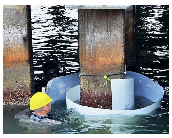
Near-Surface Mounted (NSM) Fiber-Reinforced Polymer (FRP) Jacketing
