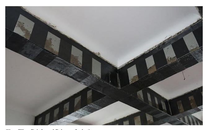
**Glass Fibre Reinforced Polymer Jacketing**
